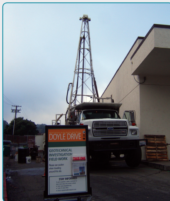
Truck mounted drill rig.
